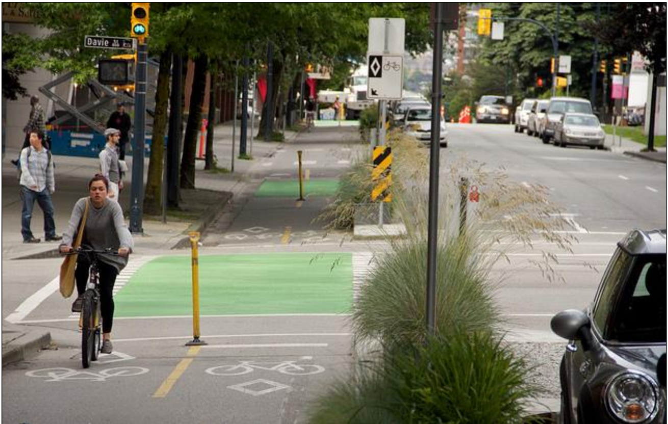
Photo of a modern, multi-modal urban street illustrating fewer lanes of traffic in favor of greater pedestrian and bicycle facilities as well as on-street parking.
