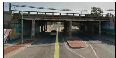
Cass Street viaduct under railroads; typical connection to neighborhoods.
