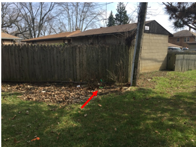
#5: Approximate Point Repair (PR) Location Looking NE at 810 Grand's backyard from 812 Grand's backyard
