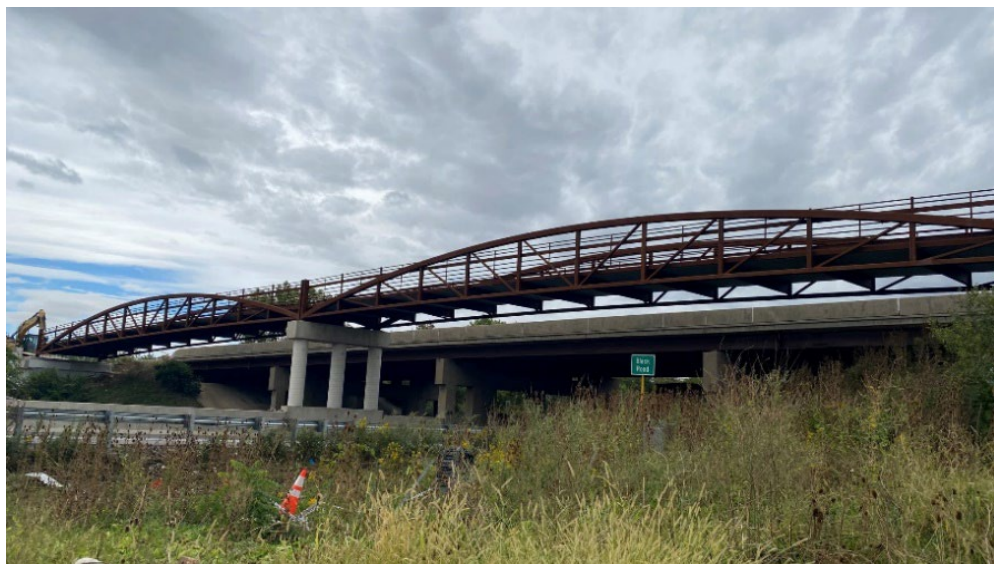
The Forest Preserve District completed the long-awaited Black Road bike bridge over Interstate 55, which established a dedicated off- road trail connection between the Hammel Woods preserve and Rock Run preserve trail systems and provides a critical link to more than 50 miles of regional trails. In addition, the Forest Preserve District continues to work on enhancing trail connections in the area, with a current focus on improvements along the Essington Road corridor.
