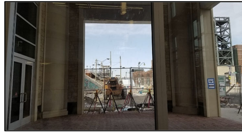
Gateway Transportation Center Under Construction
