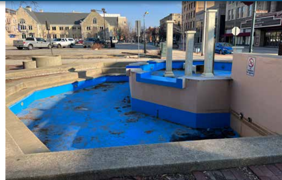
Fountain is unusable most of the year
