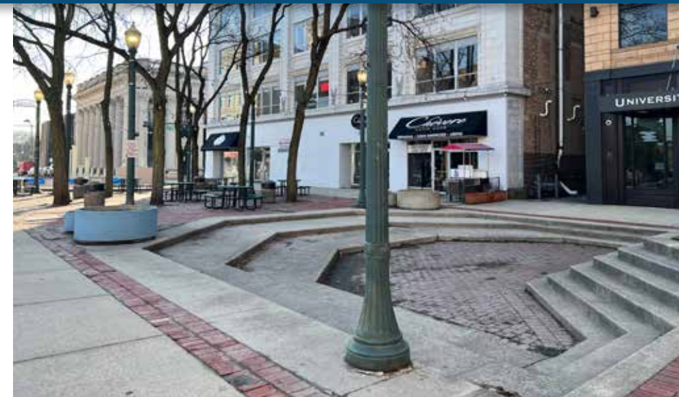
Level changes are inaccessible and create drainage problems
