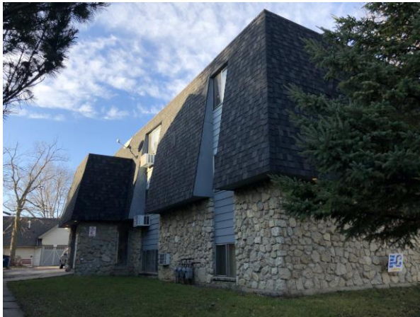
FIGURE 32: 417 N. Center Street, December 2020.
