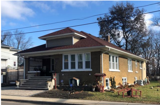
FIGURE 45: 528 N. Center Street, December 2019.
