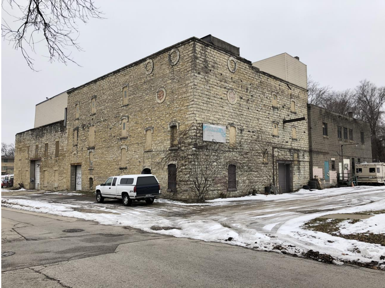
FIGURE 12: View of the extant buildings at the Scheidt & Stephens complex, January 2020.
