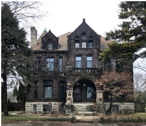
FIGURE 89: 225 N. Hickory Street, January 2020.
