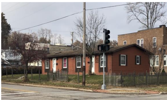
FIGURE 56: 251-253 Bridge Street, January 2020.
