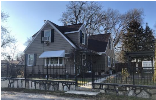
FIGURE 97: 711 Fetz Avenue, December 2019.
