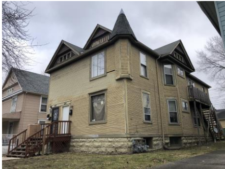
FIGURE 53: 214-216 N. Hickory Street, January 2020.
