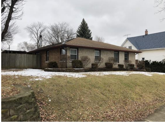
FIGURE 99: 317 Stone Street, January 2020.
