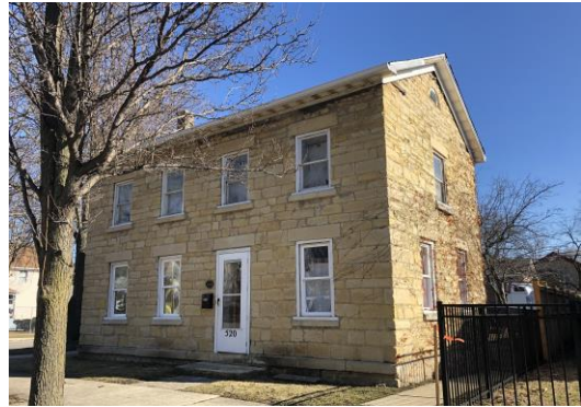
FIGURE 39: 520 N. Hickory Street, January 2020.
