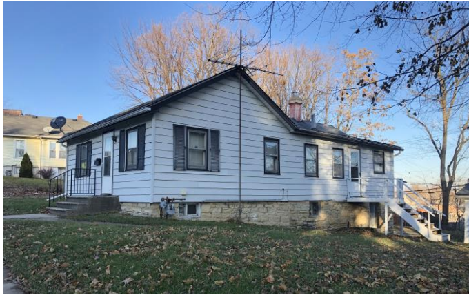
FIGURE 33: 406 N. Center Street, December 2019.
