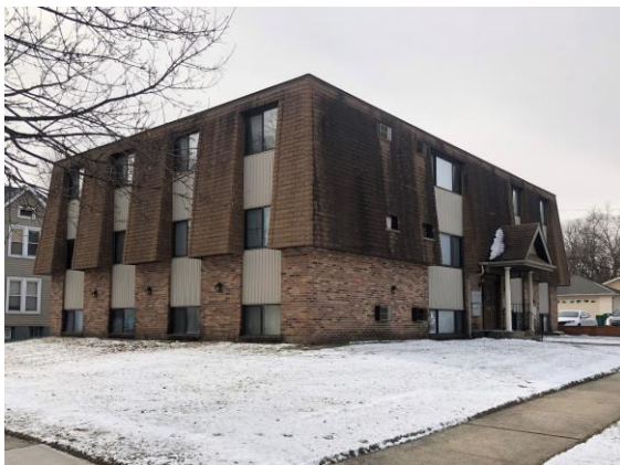
FIGURE 103: 250 Marble Street, January 2020.
