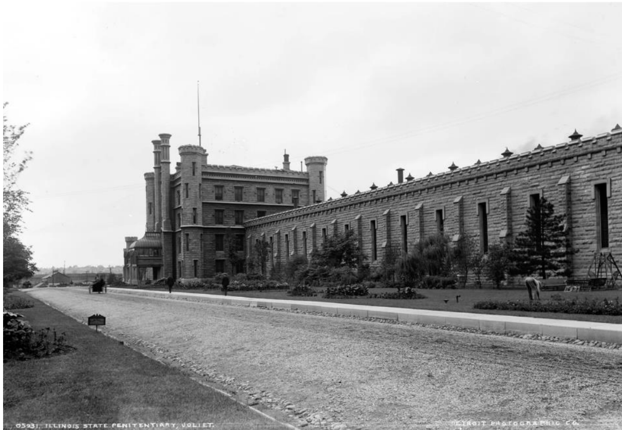
FIGURE 8: C. 1900 photograph of the Illinois State Penitentiary in Joliet Illinois by the Detroit Photographic Co.
