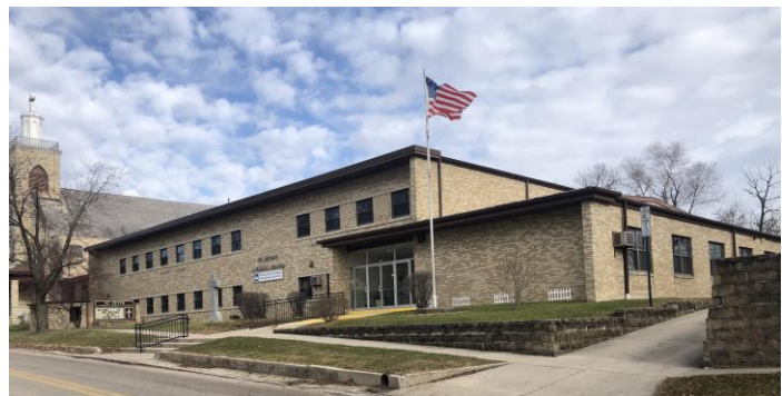
FIGURE 26: St. Peter's Lutheran School, December 2019.
