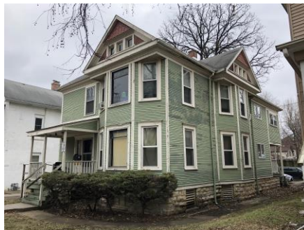
FIGURE 55: 222 N. Hickory Street, January 2020.
