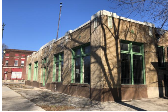
FIGURE 81: 116 N. Center Street, December 2019.
