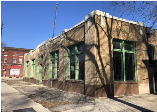
FIGURE 96: 116 N. Center Street, December 2019.
