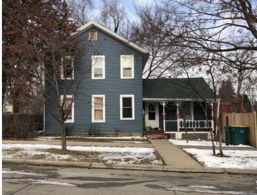
FIGURE 43: 257 Marble Street, January 2020.
