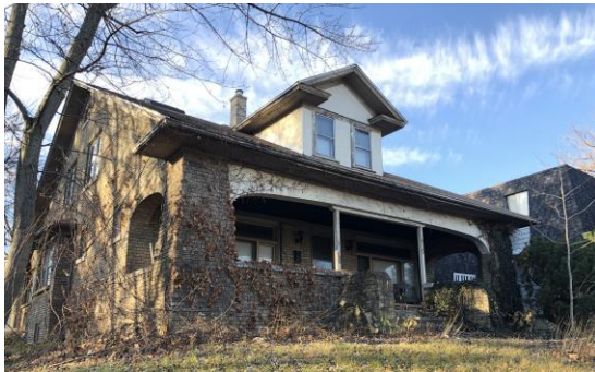
FIGURE 95: 415 N. Center Street, December 2019.
