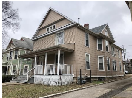
FIGURE 54: 218-220 N. Hickory Street, January 2020.
