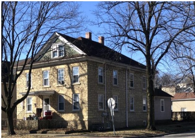
FIGURE 34: 519-521 N. Hickory Street, January 2020.
