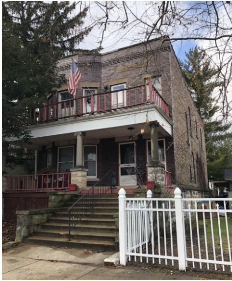
FIGURE 94: 319-321 N. Hickory Street, January 2020.
