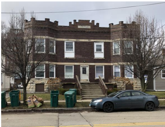
FIGURE 93: 305 N. Hickory Street, January 2020.
