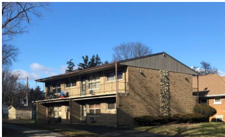
FIGURE 102: 503 N. Center Street, December 2019.
