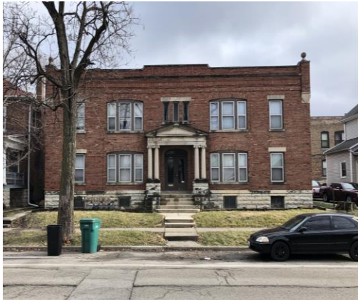
FIGURE 92: 206 N. Hickory Street, January 2020.
