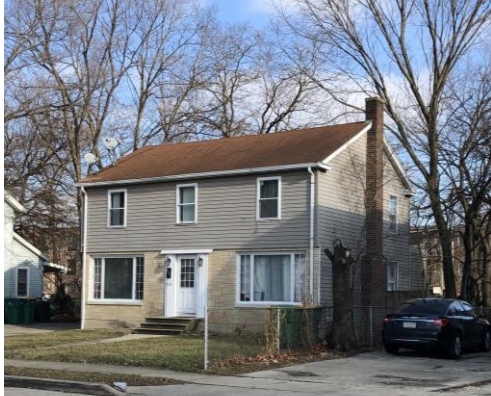
FIGURE 90: 354 N. Hickory Street, January 2020.
