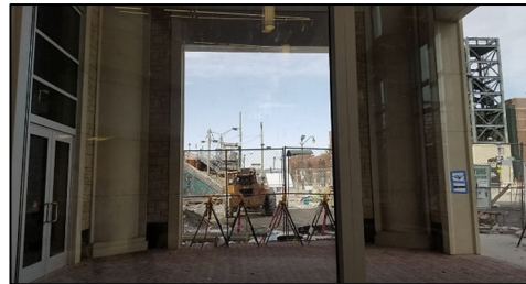
Gateway Transportation Center Under Construction
