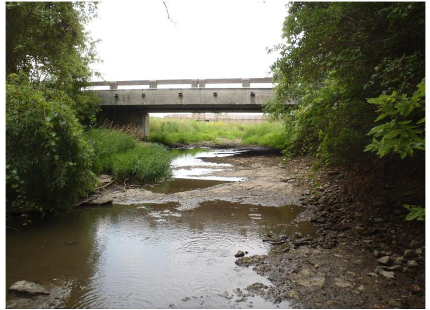
Downstream of Structure Looking Upstream (East)
