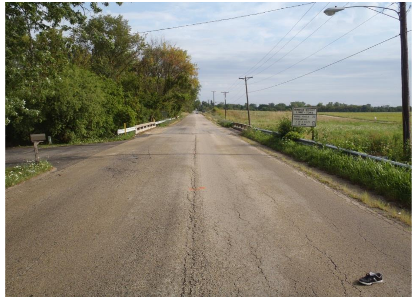
South of Structure Looking North
