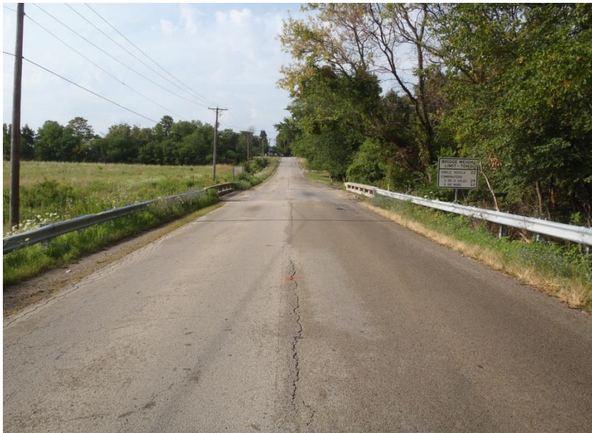
North of Structure Looking South
