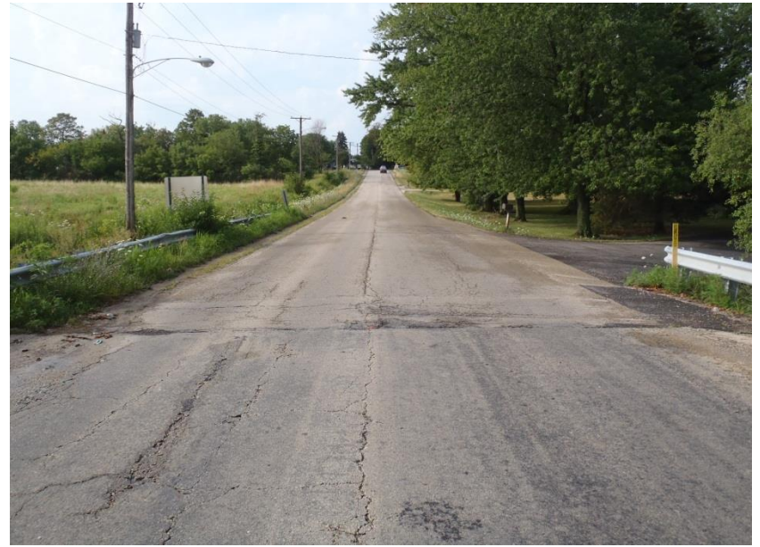
Center of Structure Looking South
