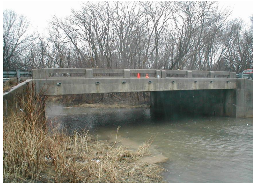
Upstream Looking at North Abutment
