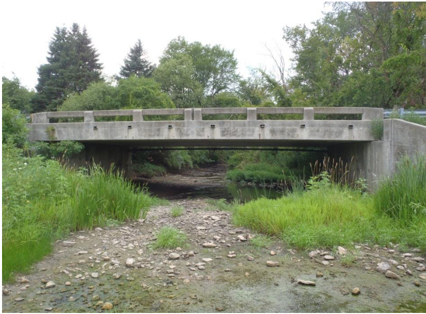
Upstream of Structure Looking Downstream (West)
