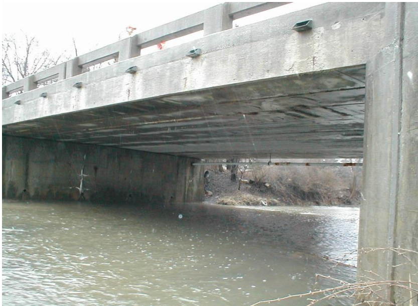
Upstream Looking at South Abutment
