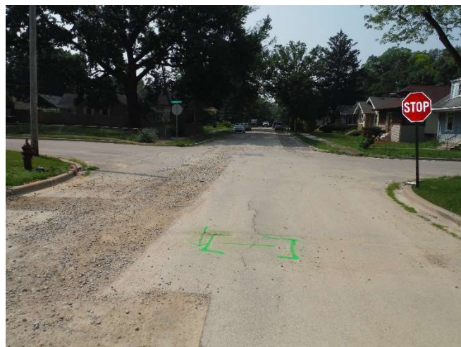
#3: Approximate PR location (Facing West)
