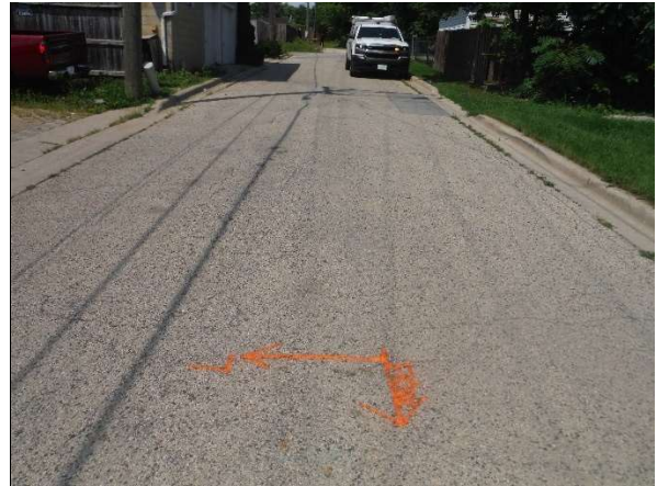
#4: Approximate PR Location (Facing West)
