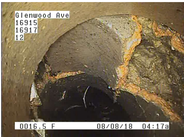
#5: Deformed Pipe
