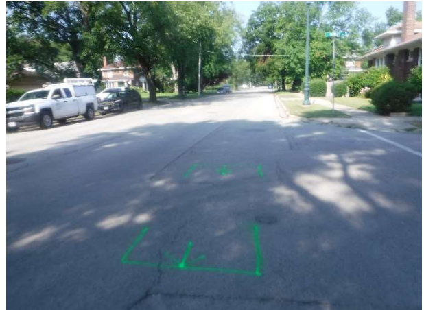
#4: Approximate PR location (Facing West)
