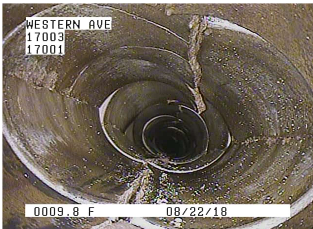
#5: Deformed Pipe
