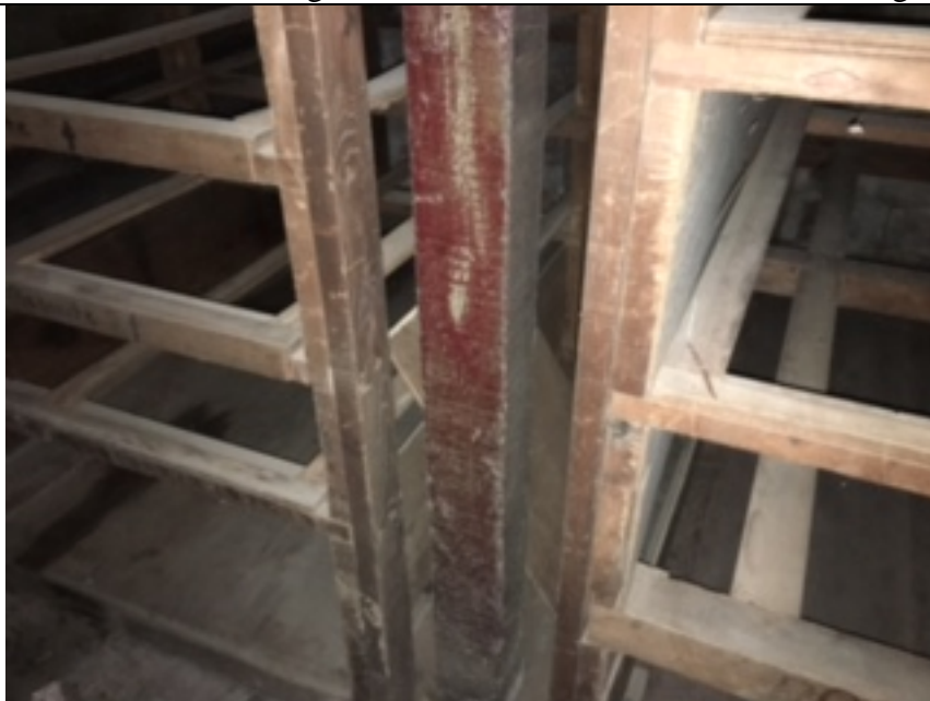
Interior NW Building 1 SE Room, Painted Wood Support Columns
