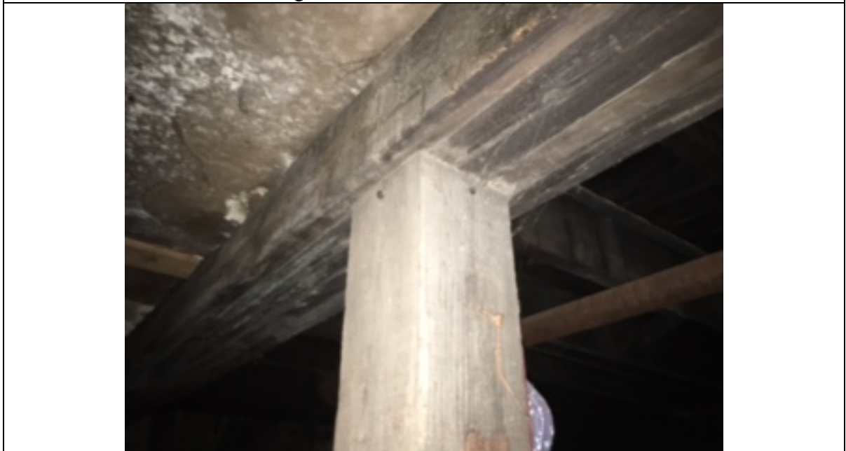
Interior NW Building Middle and South Rooms, Painted Wood Support Columns
