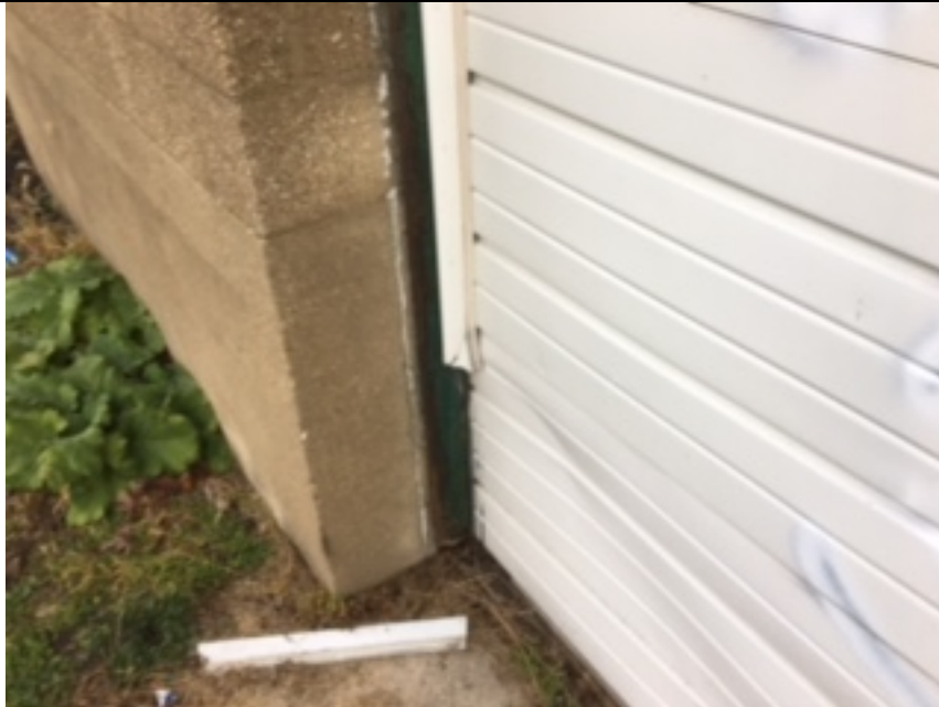
Exterior NE Building, Wall C Overhead Door Jamb (Green)
