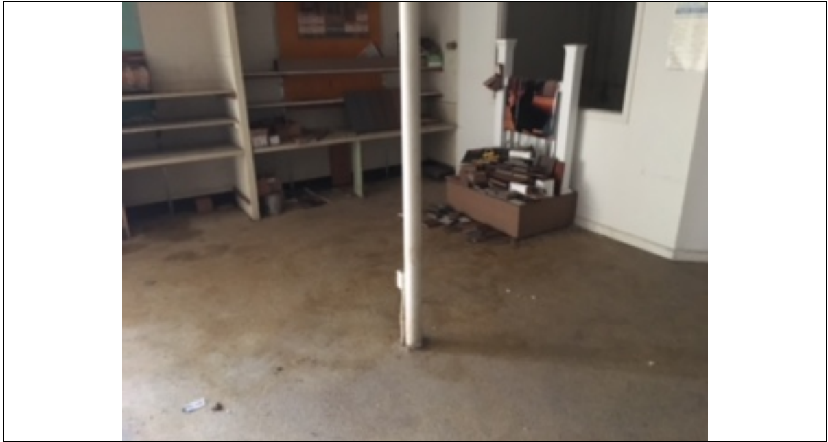
Interior NW Building, Metal Support Columns (Throughout Building)
