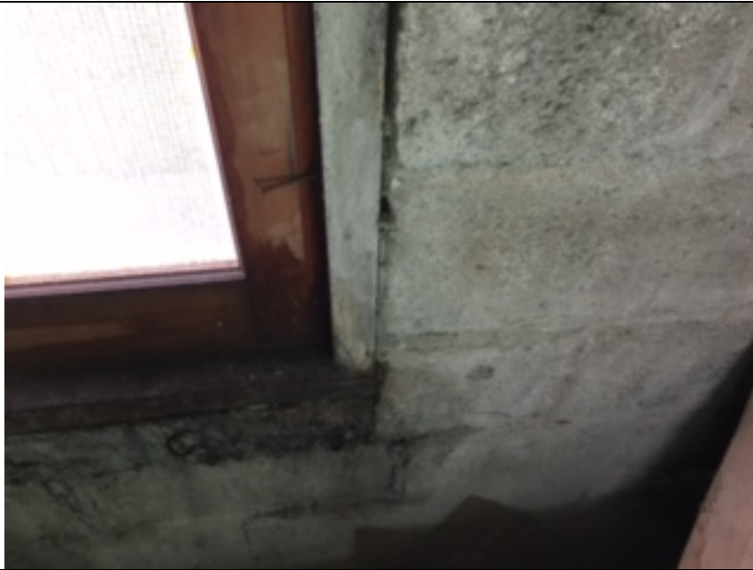
Interior NW Building 2 nd Floor, Painted Wood Window Casings
