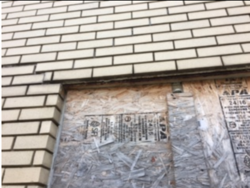
Exterior NW Building, Wall A Metal Lintel (White)
