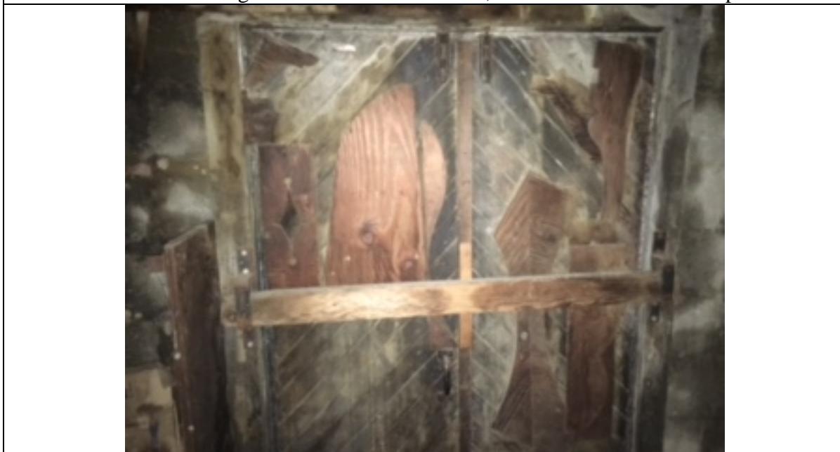
Interior NW Building SW Woodwork Room, Painted Wood Door Components
