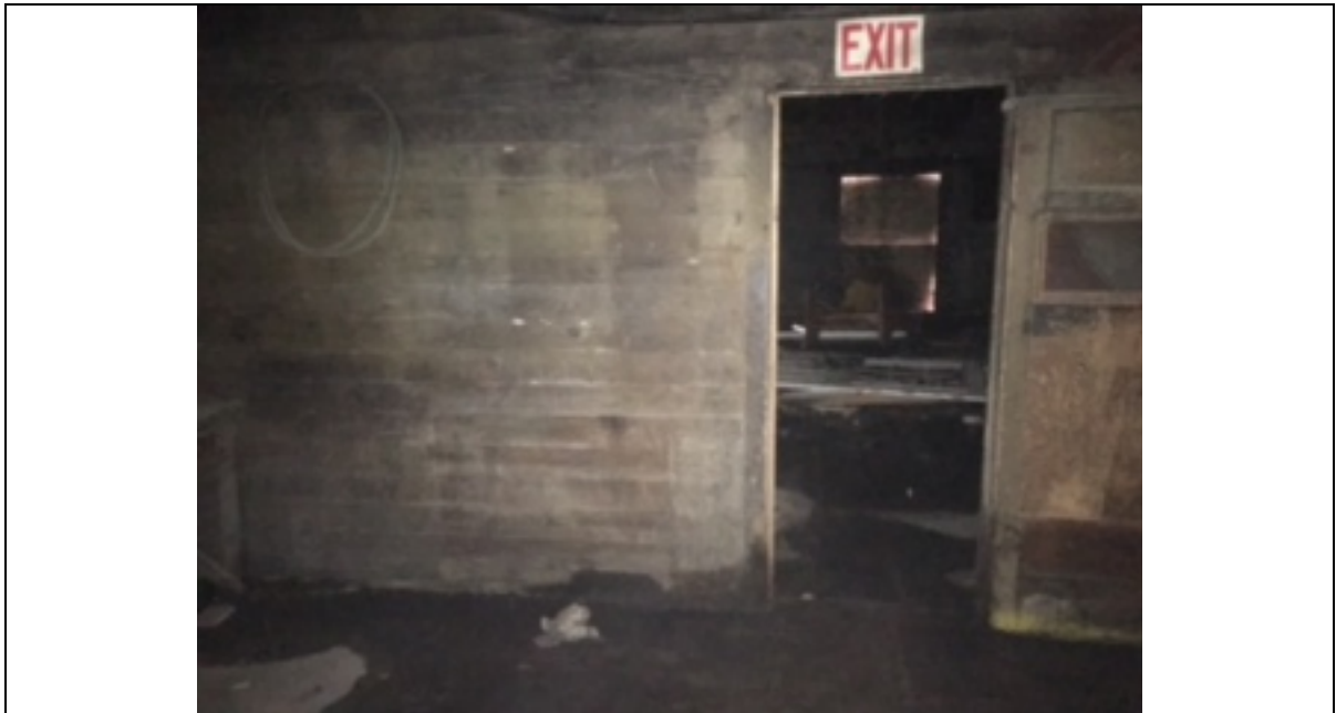
Interior NW Building Middle and South Rooms, Painted Wood Walls
