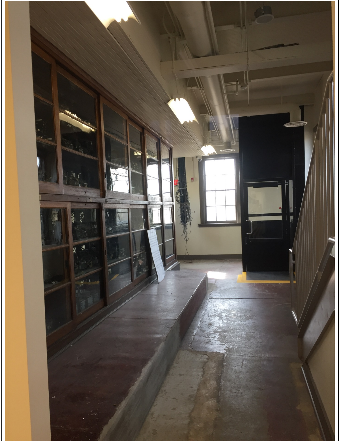
View of Relay Cabinet, Cables and Elevator
