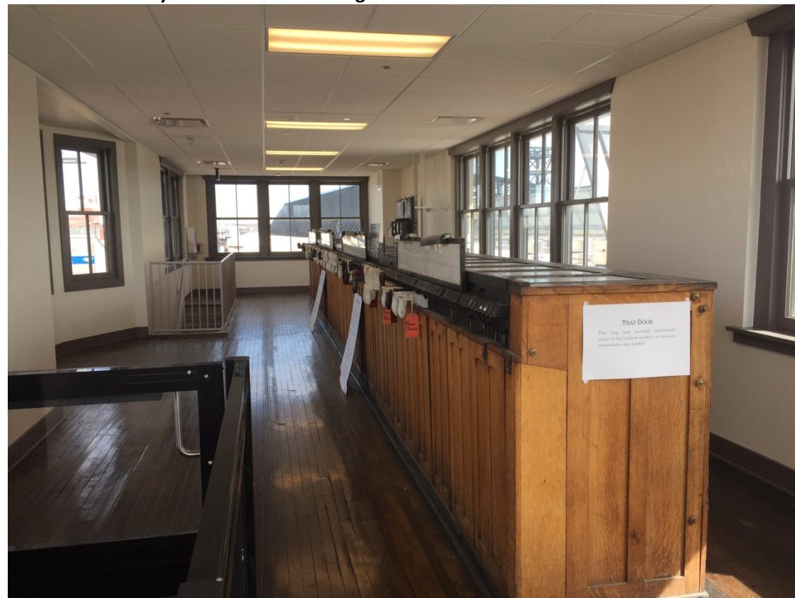
View of third story of U.D. Tower looking north.
