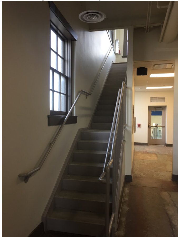
Stairs leading to the third story of U.D. Tower
