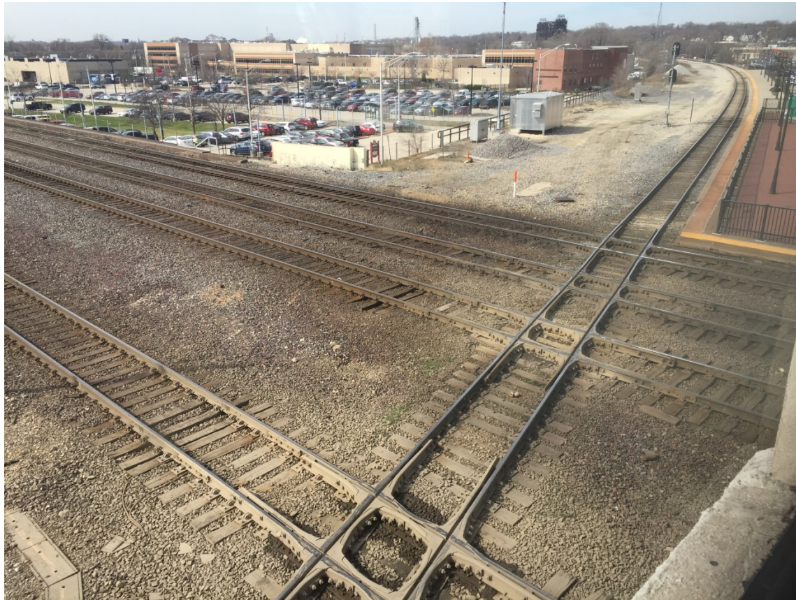
View of rail intersection from U.D. Tower.
