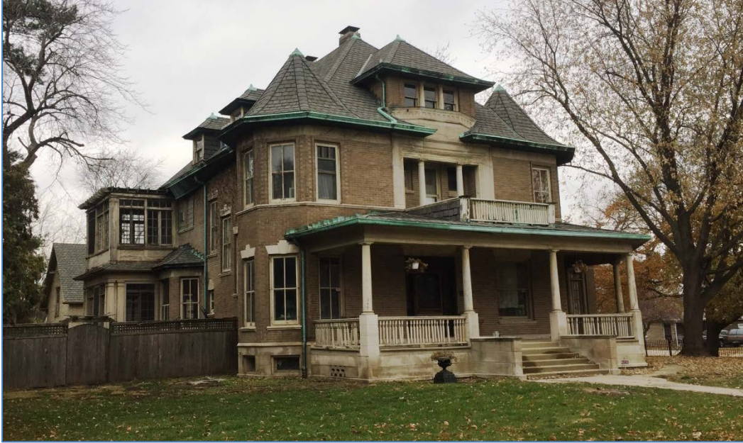
FIGURE 6: PENDING LANDMARK AT 903 WESTERN AVENUE
