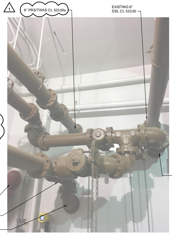
PHOTO SECONDARY DIGESTER BLDG LOOKING NORTH NTS 700-RM-2
