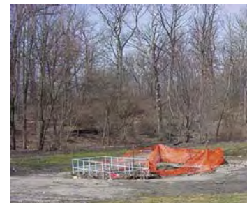
Open Utility Trench
