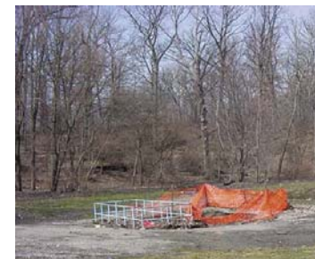
Open Utility Trench
