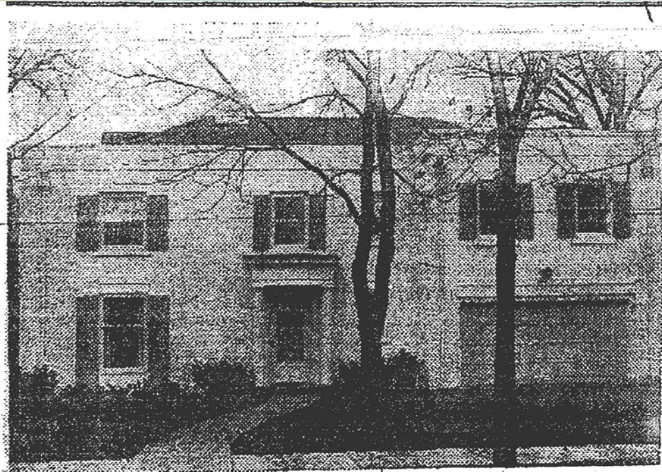
THE NINE ROOM BRICK home of Dr. and Mrs. H. V. Wadsworth, 956 Buell avenue, is of the Grecian style and it has all of the latest conveniences. Layout of the residence is such that there are maid's quarters separate from the rest of the house, a roomy study over the two car garage, three tile baths, two powder rooms, and a recreation and work room in the basement. The ceilings and walls are completely insulated. S. A. Hoberg was the contractor and A. J. Kruegel, the architect.
