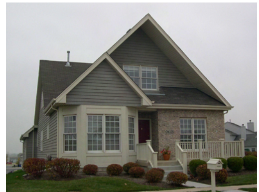
Steep Roof Pitches and Bay Windows
