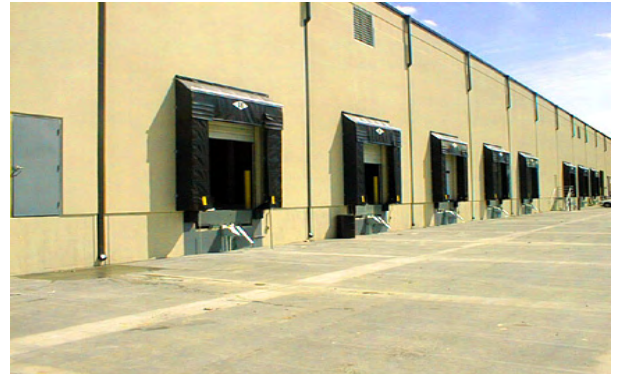
Rear Truck Loading Dock
