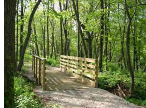
Existing Trail Through Local Forest Preserve
