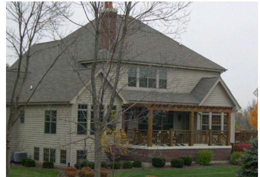
Appropriately Articulated Rear Façade as Viewed from Collector Street
